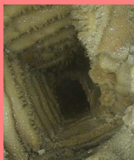
Figure 1.6 Cooling tower pack boroscope pictures
